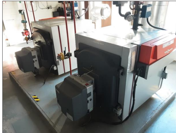
Boilers insulated with non-asbestos fibreglass.
