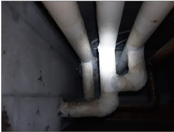
Asbestos-containing parging cement insulation on pipe elbows and tees.
