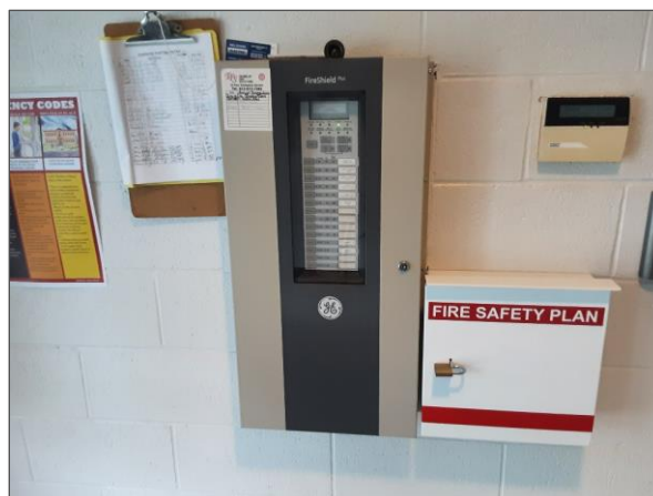
Lead-containing batteries in fire alarm control panel.
